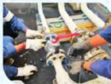
Valve Replacement & Torque Tightening
